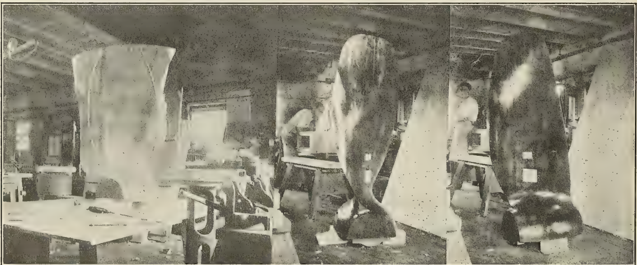
THE BLADE STANDING ON THE HUB, WITH BATTENS SPRUNG IN DEFINING BLADE EDGES. THE DIMENSIONS FOR CHECKING SHAPE OF BLADE ARE TAKEN BETWEEN THESE. THE TWO VIEWS AT RIGHT ARE OF THE COMPLETED PATTERN OF ONE BLADE.
